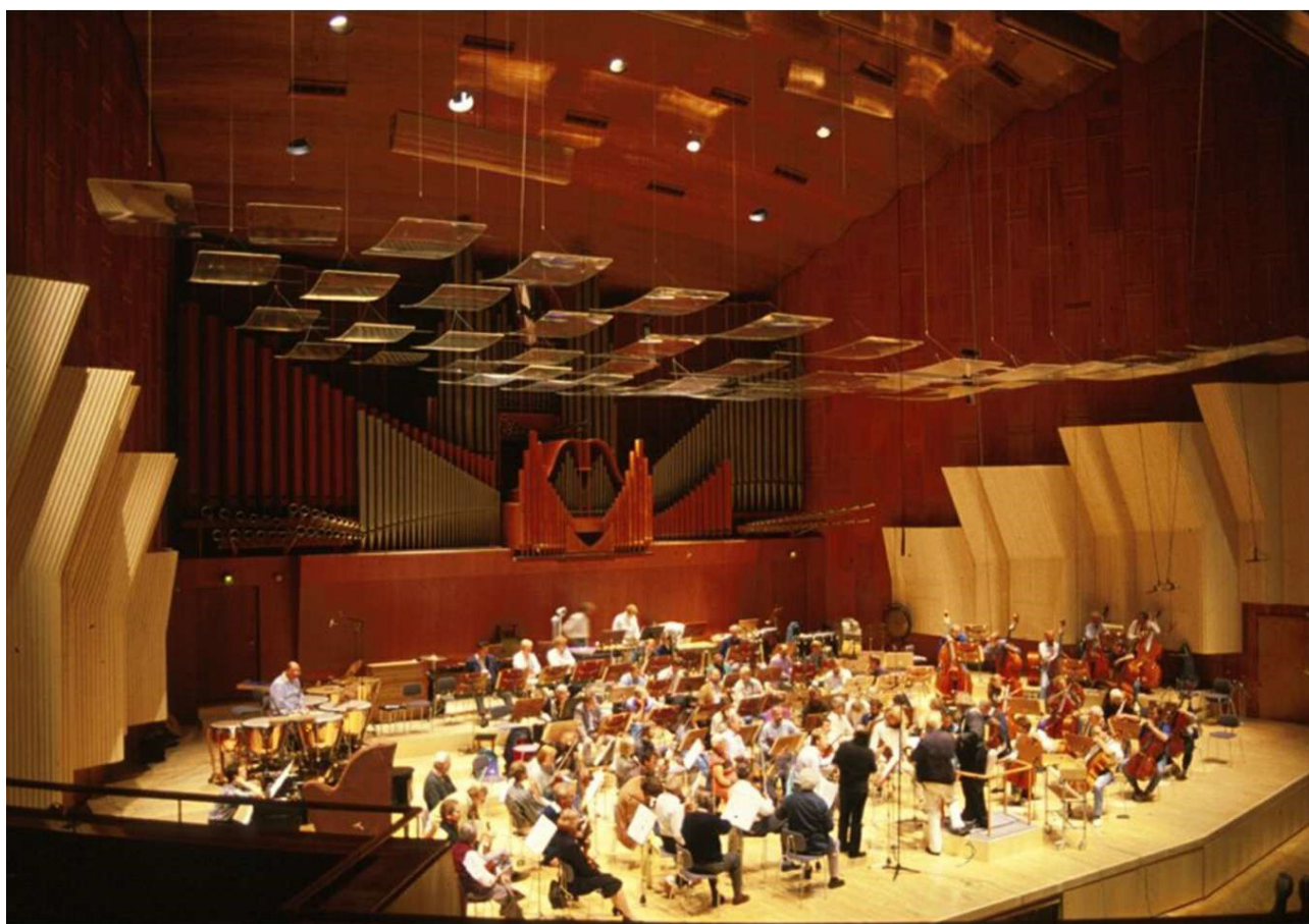
Fig. 11: Photo from the concert hall after the new reflector array and new wall reflectors were installed in 1989.
