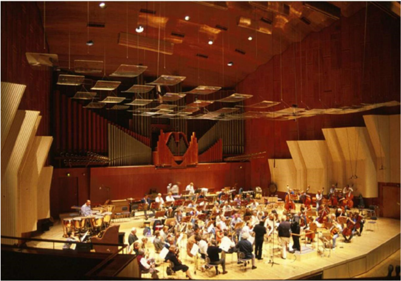
Figure 11: Photo from the concert hall after the new reflector array and new wall reflectors were installed in 1989.
