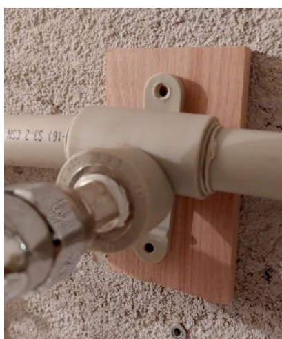
Fig. 4: Methods of the wall elbow fixing – wooden support with screws (left), wooden support without screws (centre), without fixing the wall elbow (right).
