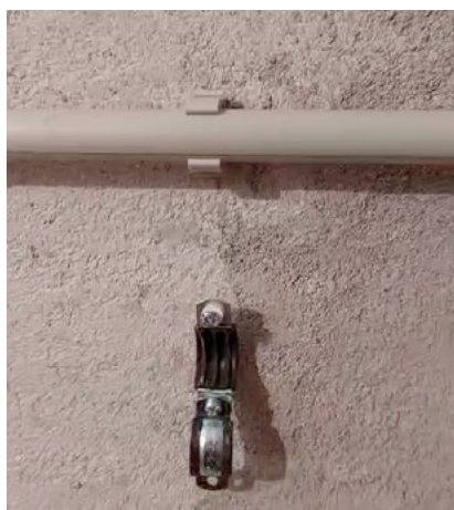
Fig. 3: Methods of pipe fixing – PPR clamps (left), rubber lined clamps (centre), free hanging pipe (right).
