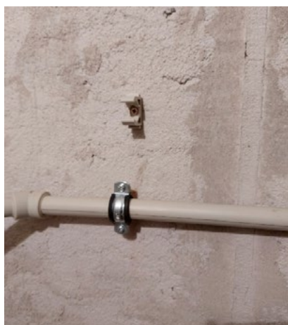
Fig. 3: Methods of pipe fixing – PPR clamps (left), rubber lined clamps (centre), free hanging pipe (right).
