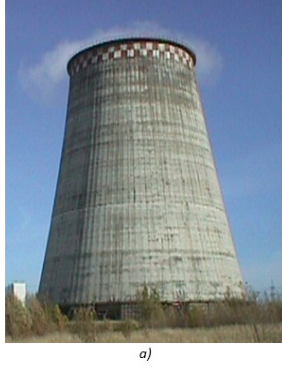
Fig. 1: Natural draft counterflow cooling towers: a — construction; b — intake windows
